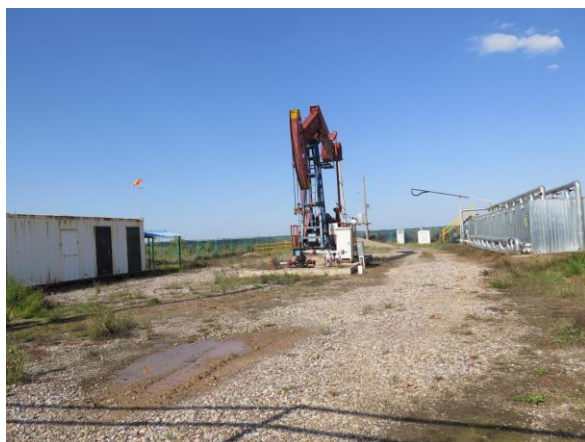
场地碎石压盖 (17P7 井场)
